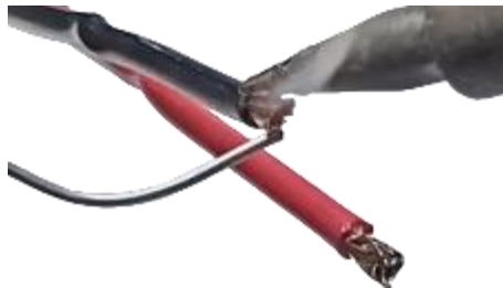
Begin to solder both cables
